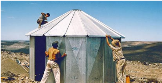
Fig. 13: Ample use was made of “rondavel”-type of temporary buildings which could easily be erected and broken down again, particularly handy in the mountainous terrain of the Nieuwveld plateau. Credit: ESO, J Doornenbal
