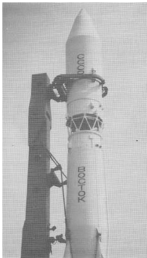
Fig. 2 (left) Vostok 1 on top of the modified ICBM R-7 rocket, prior to launch on 12 April, 1961.
