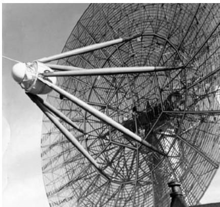
The TLM-18 60 foot automatic tracking antenna showing the feed support and arms. This was situated at Fort Monmouth, New Jersey.
