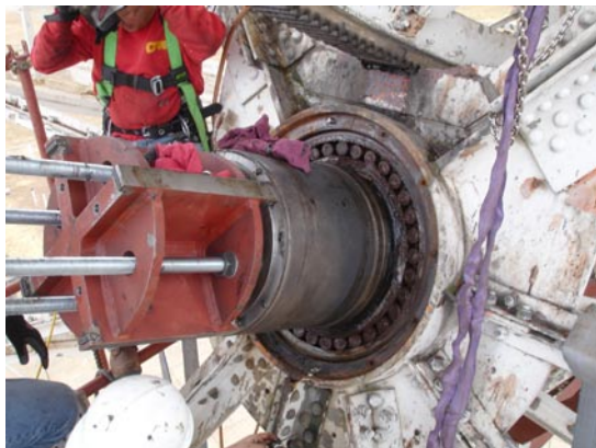
Fragments of broken bearing fell out when the south polar shaft bearing got exposed.
