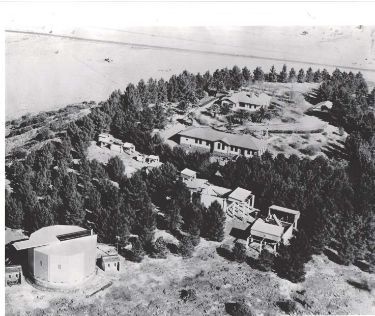
Fig 4. Boyden Observatory in 1952, with all the domes opened and the telescopes proudly "exposed" for the camera. Source: Friends of Boyden.
