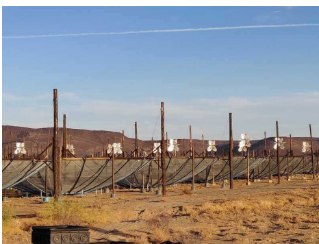
Fig 5. Side view of the HERA array. The dish surface is constructed of wire birdcage netting and supported by ordinary PVC tubing and fittings.
