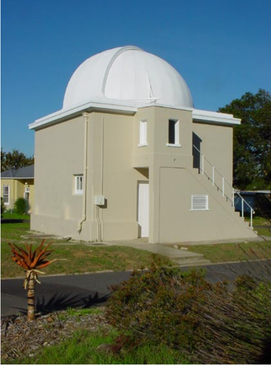
Fig. 7. The Astrographic building and dome (May 2012), just after repainting and exterior renovation.
