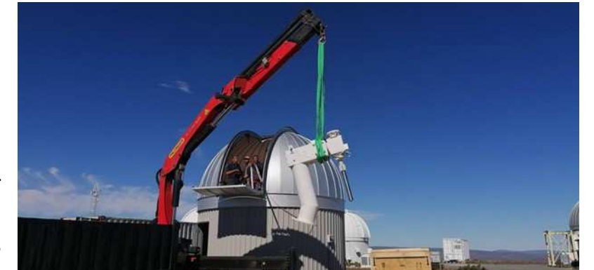
Fig 1. The Sutherland ATLAS station during construction in South Africa. Photo: Willie Koorts/SAAO
