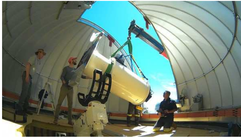
Fig 2. SAAO Staff installing ATLAS-Sutherland. (Left: Willie Koorts, Centre: Nic Erasmus, Right: Crane Operator) Photo: Willie Koorts/SAAO.
