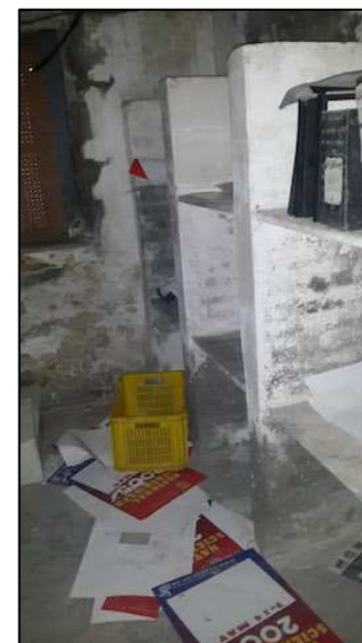
Fig 6. Part of the West basement, Main Building.
