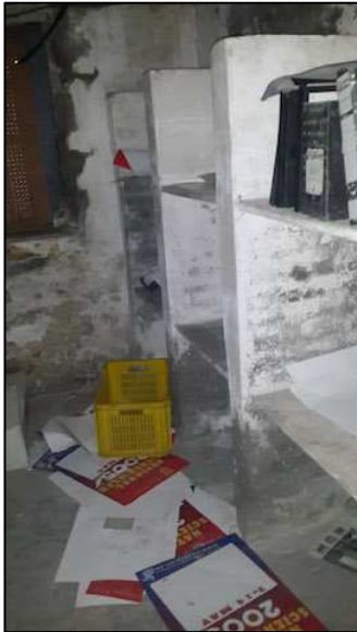
Fig 6. Part of the West basement, Main Building.
