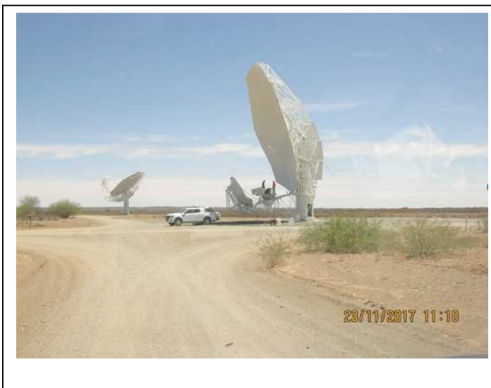
Fig 2. One of the 64 Offset Gregorian dishes that make up the MeerKAT
