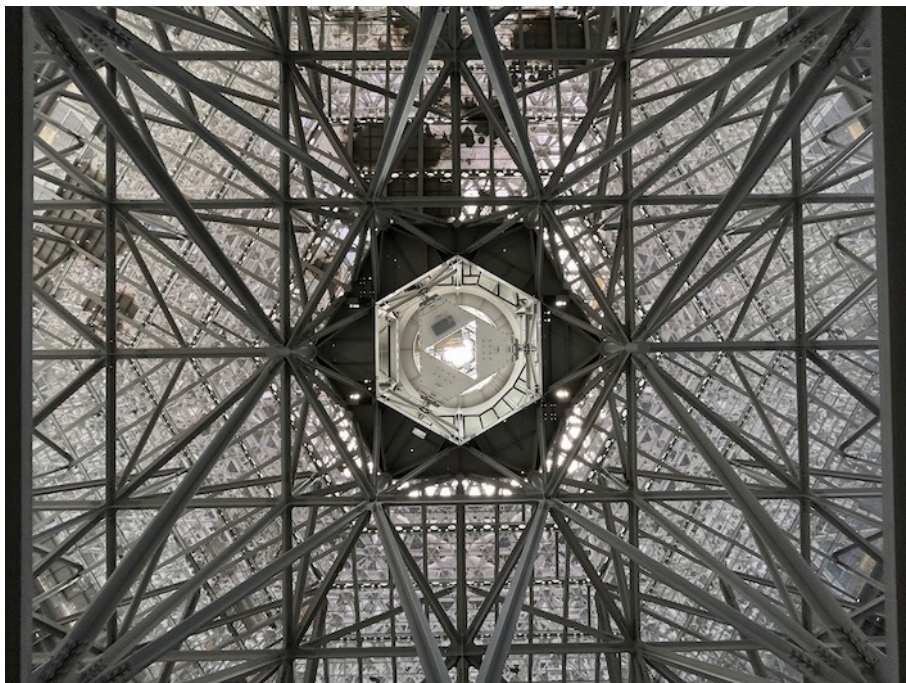
Fig 8: Looking up through the ELT primary mirror truss from below, to where the optical tower will house M2, M3 & M4.
