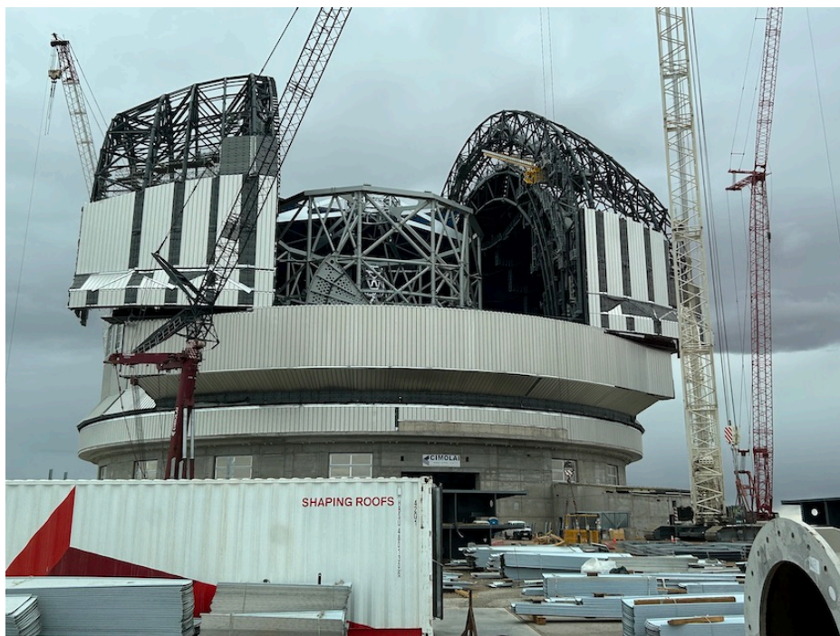
Fig 6: ELT enclosure under construction, with the telescope structure visible inside & the dome shutters being completed.
