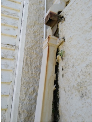
Figs 8, 9: (left and centre) Original cast iron drain pipes becoming detached from wall. Mould growing on wall and weeds rooting in wall.
