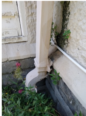
Figs 8, 9: (left and centre) Original cast iron drain pipes becoming detached from wall. Mould growing on wall and weeds rooting in wall.
