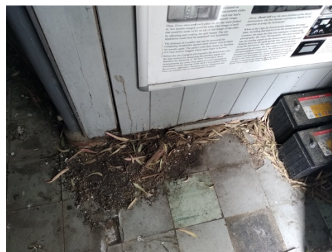
Figs 18 & 19: The interior of the building, showing the result of bird invasion and leaks.
