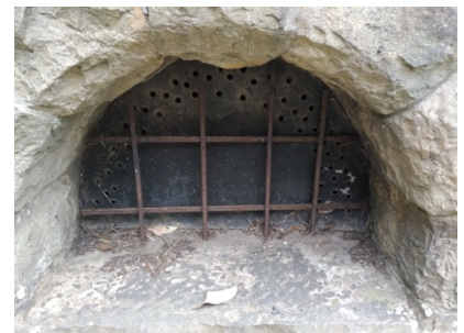
Fig 11: The grills over the basement windows are loose and will not deter any determined intruder.
