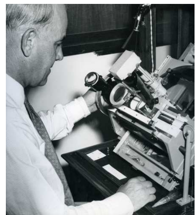
Fig 9. Hilger 2-coordinate measuring machine (SAAO Museum Cat. # M182).
