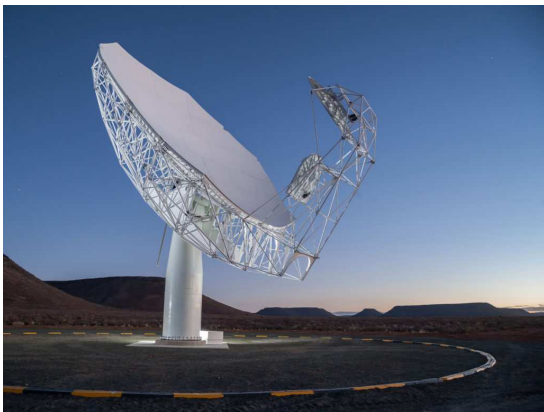
Fig 4. A single MeerKAT antenna. The radio signals bounce off the big dish onto the smaller one at right and then into the receiver just below the small one (Photo: SARA0).
