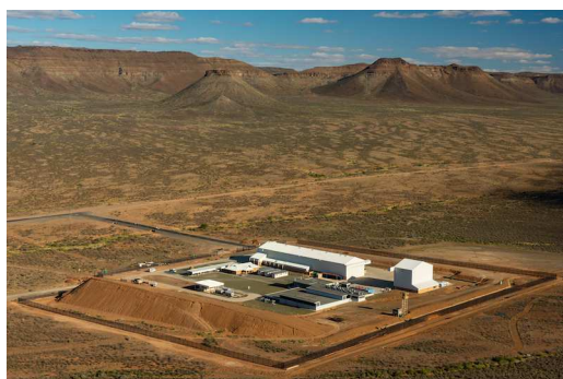
Fig 12. The support buildings at the SARAo site, including the Karoo Array Processor Building where powerful computers assemble the signals from the individual antennas (Photo: SARAo).
