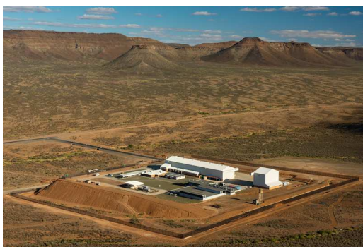
Fig 12. The support buildings at the SARAO site, including the Karoo Array Processor Building where powerful computers assemble the signals from the individual antennas (Photo: SARAO).
