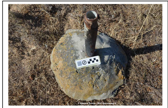
Fig 2. What appears to be the base of a later Trig Beacon that had fallen off.
