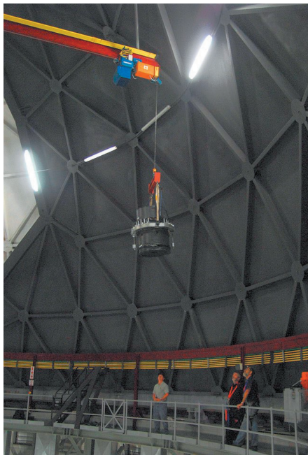
The SAC being lowered by the dome crane. Picture: Lisa Crause
