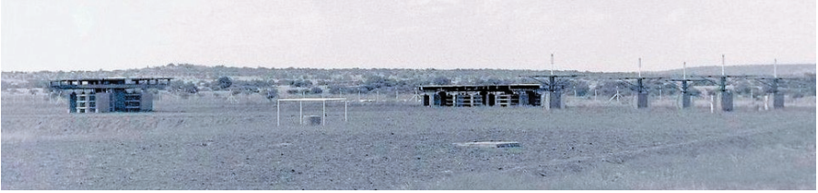
Part of the DIANE interferometer (the French equivalent of the United States MINI-TRACK). This operated in the 136-138 Mhz radio frequency band and was used to determine the orbit of a satellite using the satellites onboard radio transmitter. Picture: Greg Roberts, Easter 1966.
