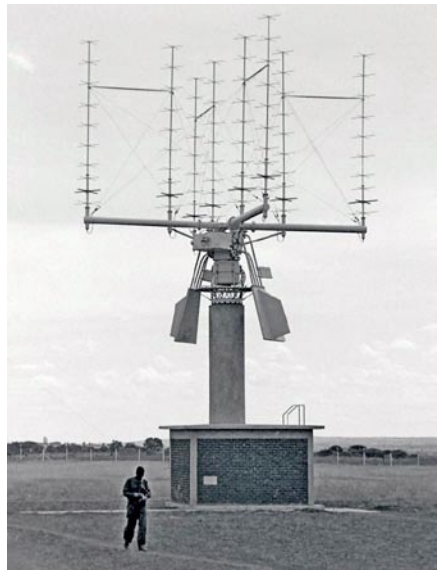
The IRIS antenna – a large array of eight cross-axis yagi antennas used to receive telemetry from satellites operating in the 136-138 Mhz radio band. In addition, commands could be transmitted to the satellite on a frequency close to 148 Mhz. The entire array could be moved in azimuth and altitude to any part of the sky and could follow the satellite as it passed over the station. Picture: Greg Roberts, Easter 1966.
