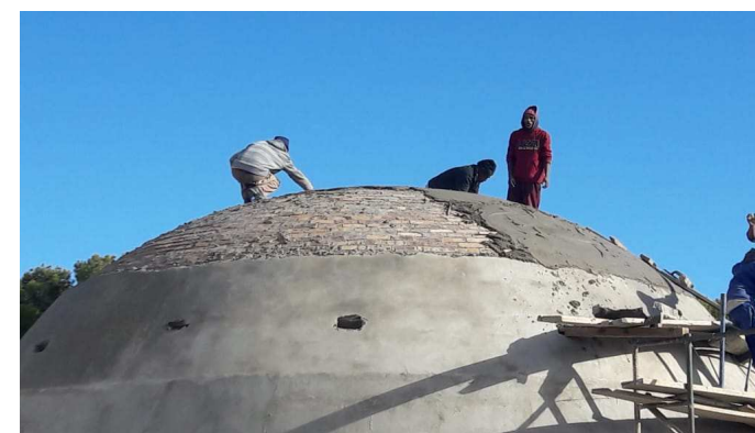
Fig 9: Plastering the outside of the dome.
