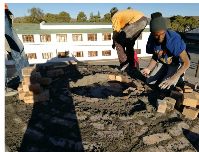
Fig 8: Nearing completion of the brickwork
