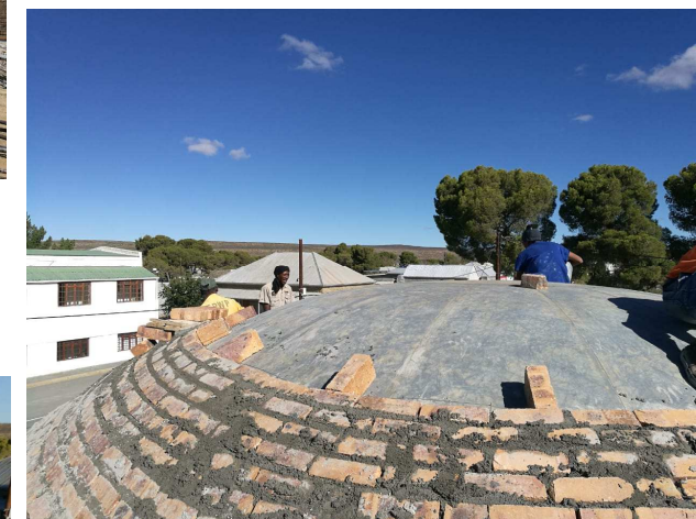
Fig 8: Nearing completion of the brickwork
