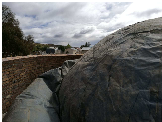
Fig 5: The deflated balloon placed inside the walls.
