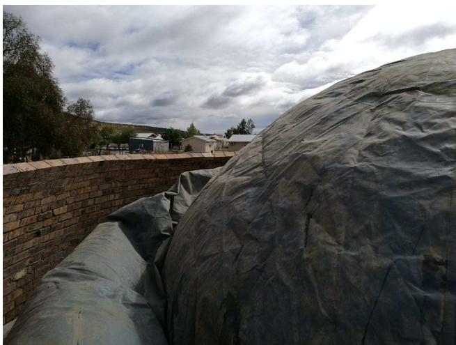
Fig 5: The deflated balloon placed inside the walls.
