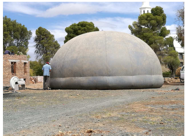
Figure 4. The inflated balloon to be used as a "mould" outside the walls.
