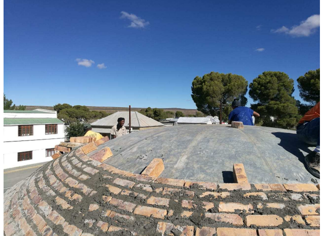
Fig 8: Nearing completion of the brickwork
