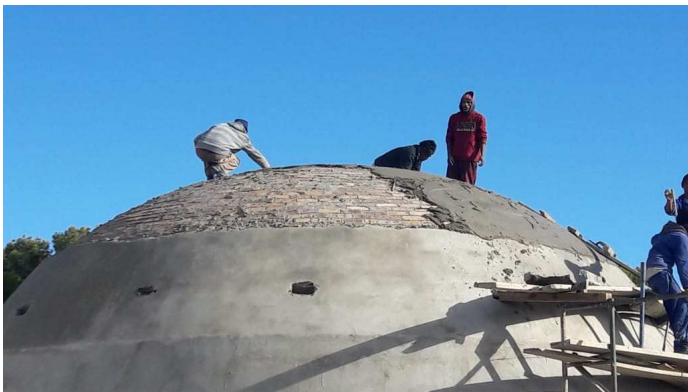
Fig 9: Plastering the outside of the dome.
