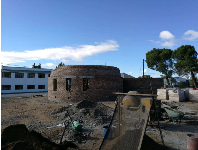
Fig 3: Base walls with the first 1.5 m curved wall.
