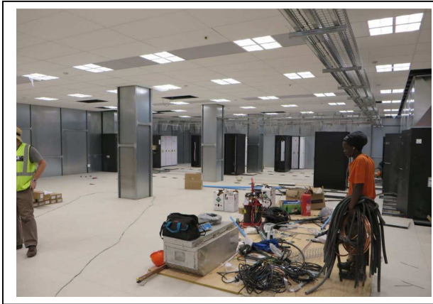
Fig 1. Final touches being applied to the RFI-shielded room in the Karoo Array Processor Building.
