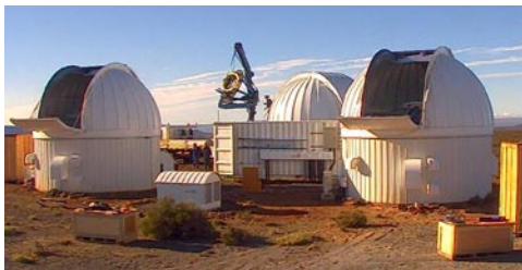
Only 45 minutes after the first one, the third telescope was carefully guided through its dome-slit by engineer Annie Hjelstrom.
