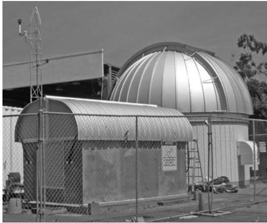
A full size Aqawan in the foreground with the 5.6m diameter Ash Dome behind it, seen here deployed in the LCOGT headquarters car park for testing. (Source: LCOGT)
